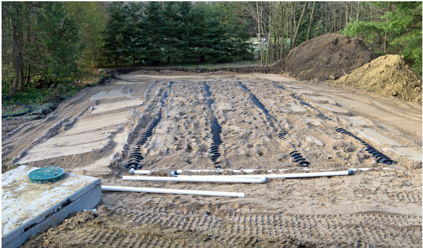
Figure 11: Example of septic system installation.
